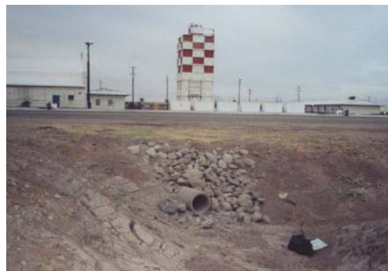
Figure 5. A pair of burrowing owls used this culvert under taxiway D in 2003.
