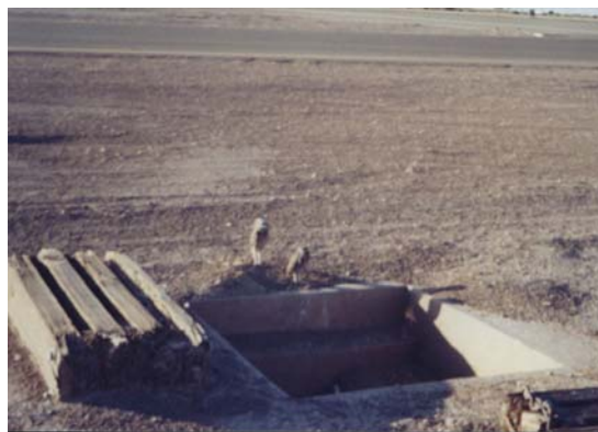
Figure 9. Opened structures such as this wire conduit access point can provide shelter to burrowing owls. Photo: J. A. Gervais
