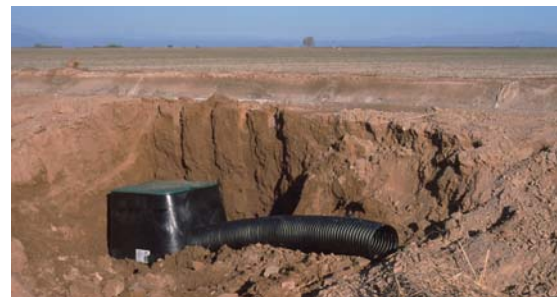
Figure 13. An artificial burrow under construction. Photo: D. K. Rosenberg
